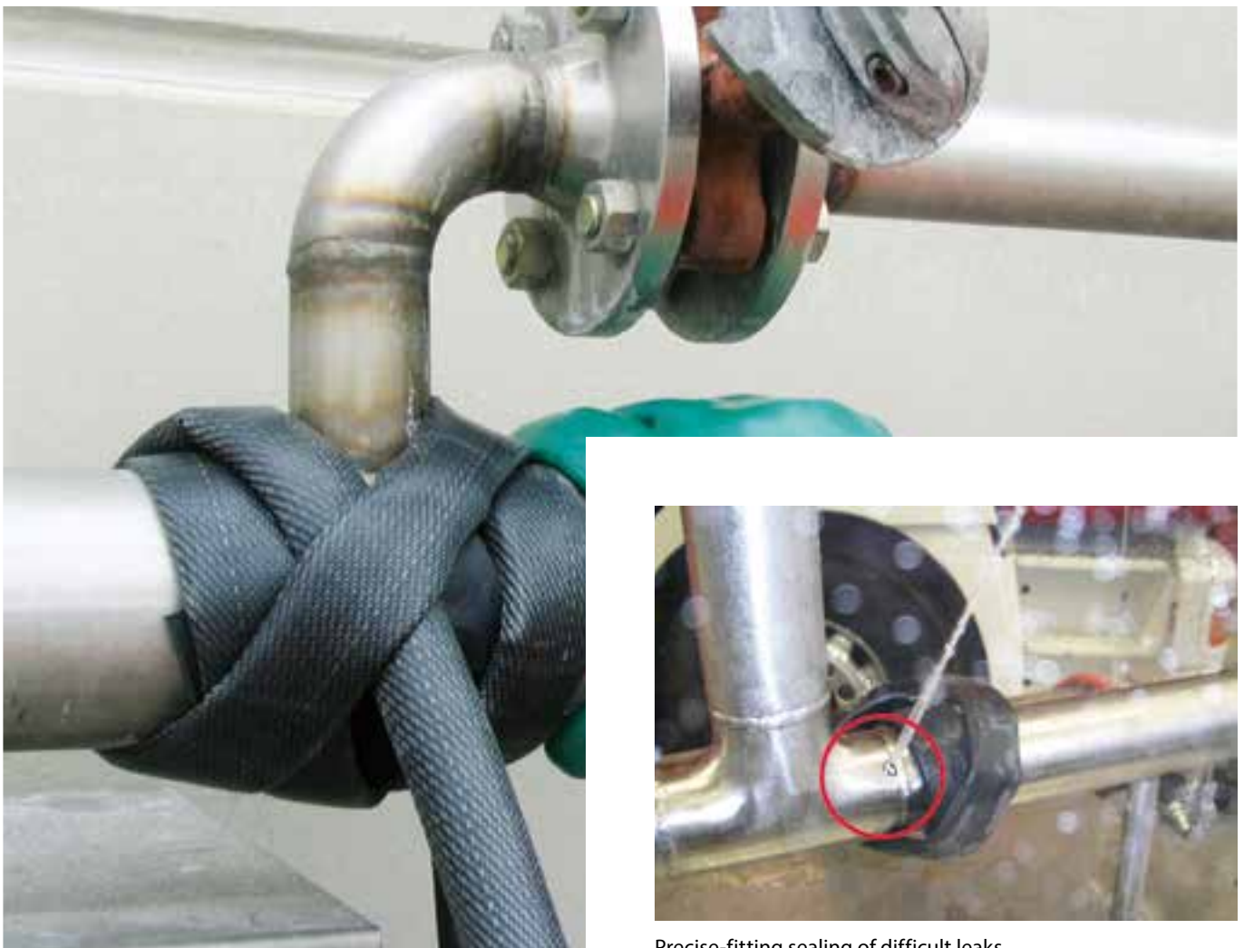
Precise-fitting sealing of difficult leaks
